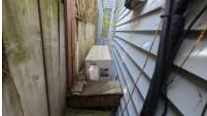
Pic. 4: AC compress – should be levelled
