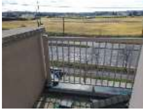
Pic. 13: 3rd floor balcony
