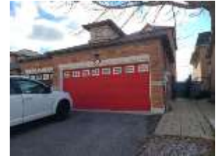
Pic. 4: Detached garage
