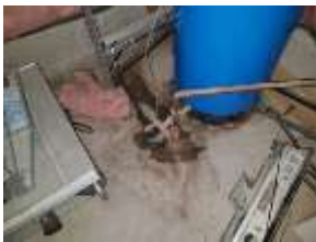
Image 37: Small water leak at well pump
