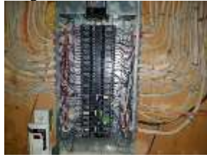
Image 42: 200 amp breaker panel with all copper wire
