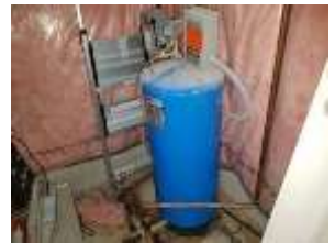
Image 36: Well pressure tank
