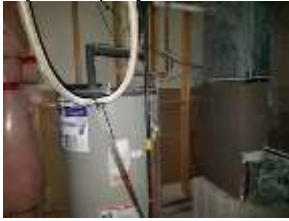
Image 41: Electric water heater
