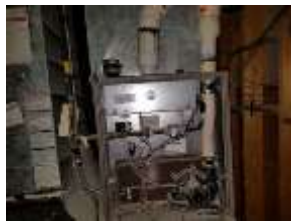
Image 38: High efficiency gas furnace
