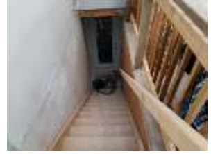
Image 4: Basement entrance via garage
