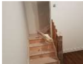
Image 35: Unfinished basement stairs
