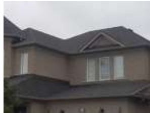
Pic. 2: New roof covering
