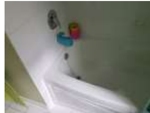
Pic. 15: 2 nd floor bath
