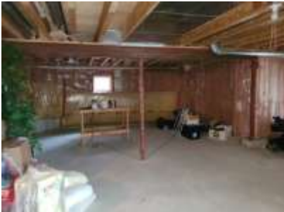
Pic. 25: Unfinished basement
