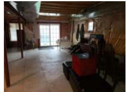
Pic. 24: Unfinished basement
