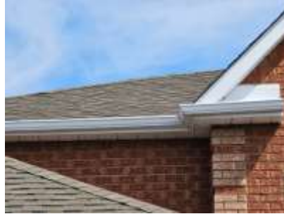
Pic. 2: Updated roof covering
