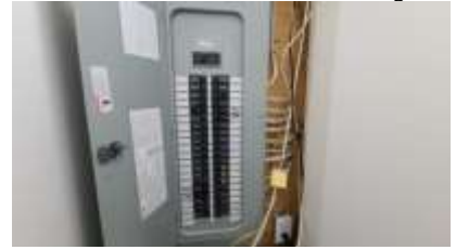
Pic. 42: 200 amp breaker panel
