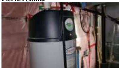
Pic. 38: Hot water tank 2015
