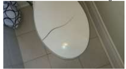
Pic. 21: Cracked toilet seat
