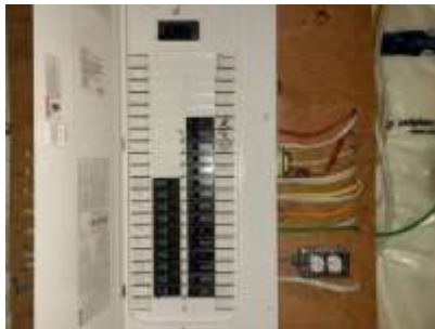
Pic. 29: 200 amp breaker panel
