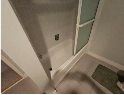
Pic. 31: Basement bath
