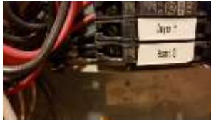
Pic. 41: Double tapped breaker
