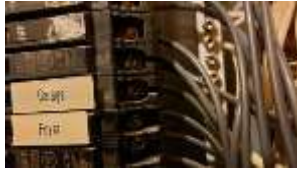
Pic. 42: Double tapped breaker
