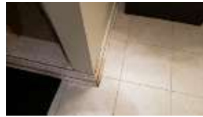
Pic. 35: Water damage outside shower
