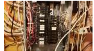
Pic. 40: 100 amp breaker panel
