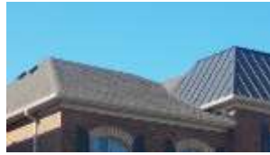
Pic. 2: Roof covering
