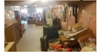
Pic. 28: Unfinished basement
