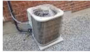
Pic. 3: AC unit
