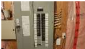
Pic. 34: 200 amp breaker panel with all copper wire
