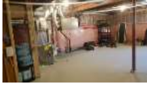
Pic. 30: Unfinished basement
