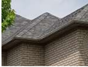
Pic. 2: Updated roof covering
