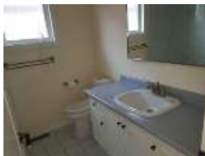
Pic. 14: 2 nd floor bath
