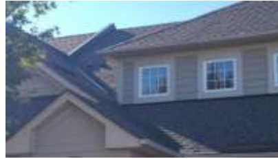
Pic. 2: Roof covering
