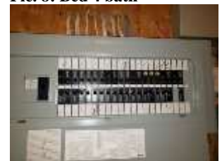
Pic. 12: 200 amp breaker panel
