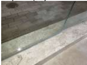
Pic. 25: Shower wall loose at the bottom
