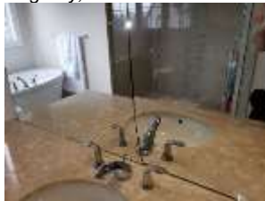
Pic. 26: Cracked mirror in master bath
