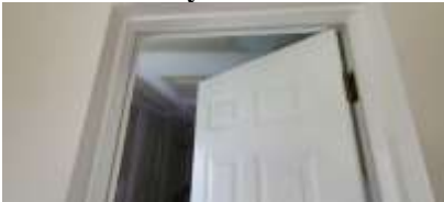
Pic. 7: Garage entry door has no auto closer and opens into the garage onto steps
