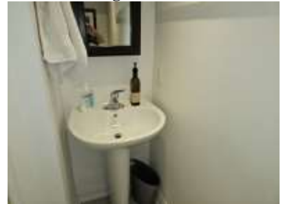
Pic. 27: Basement bathroom
