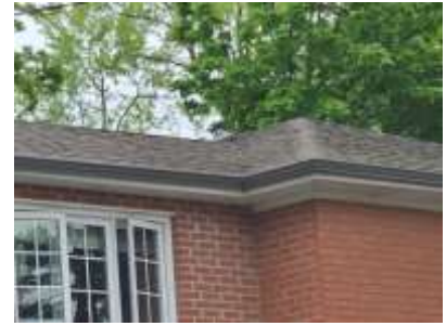
Pic. 3: Updated roof covering
