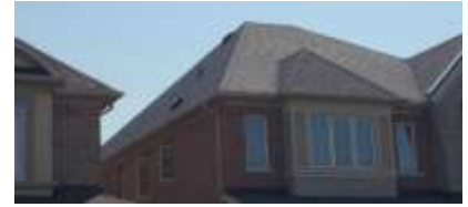
Pic. 3: Original roof covering
