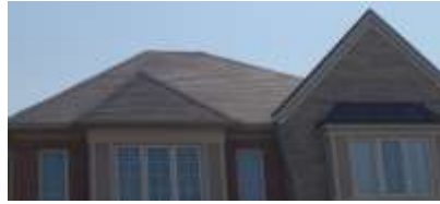
Pic. 2: Original roof covering
