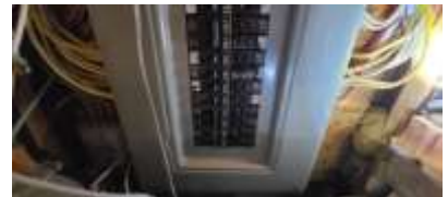
Pic. 36: 200 amp breaker panel
