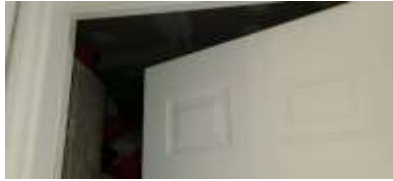
Pic. 26: Garage entry door no auto closer
