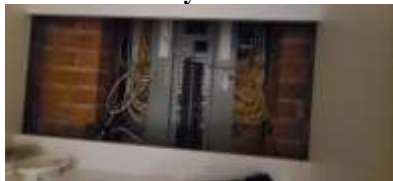
Pic. 35: 200 amp breaker panel
