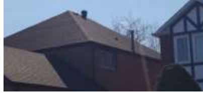
Pic. 2: Updated roof covering
