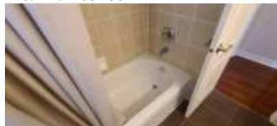
Pic. 14: 2 nd floor bath
