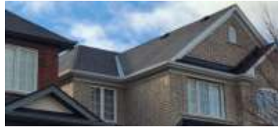
Pic. 2: Updated roof covering
