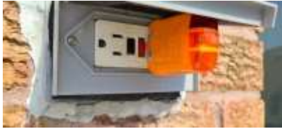
Pic. 4: Rear GFCI won't trip – needs replacement
