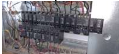
Pic. 26: 50% copper 50% aluminum wiring, bonding reviewed was all correct
