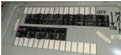
Pic. 25: 100 amp breaker panel
