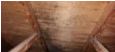
Pic. 7: Minor amount of surface mould likely caused by the improper bathroom exhaust vent pipe
