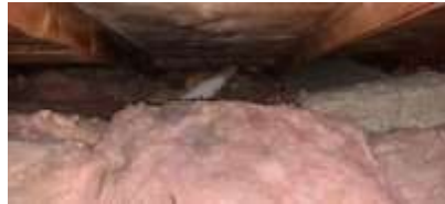
Pic. 8: Recommend upgrading the bathroom exhaust vent pipe to an insulated pipe
