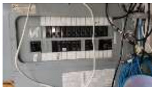
Pic. 26: 100 amp breaker panel
