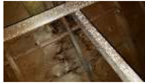
Pic. 7: Old water marks in attic – all dry
