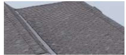
Pic. 3: Original roof covering
