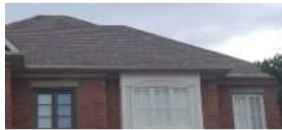
Pic. 2: Original roof covering
