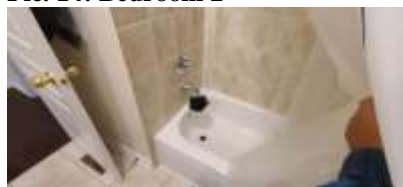
Pic. 17: 2nd floor bath
