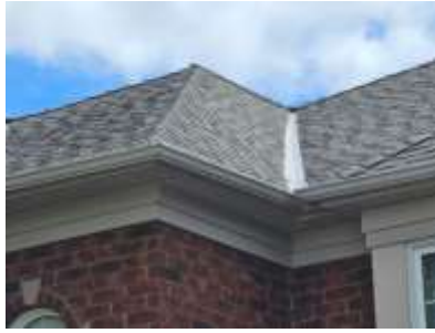
Pic. 2: Updated roof covering
